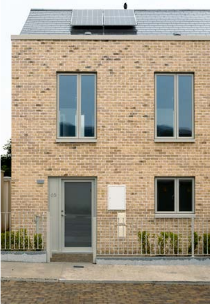
Example of ESB meters on front facade
